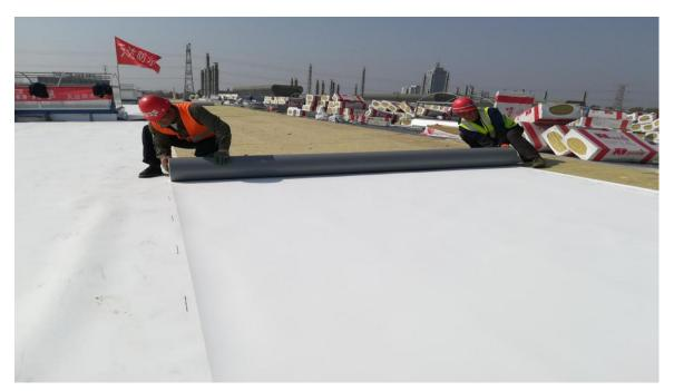
A:Roofing waterproofing membrane –suitable for low slope applications (new construction or renovation)
